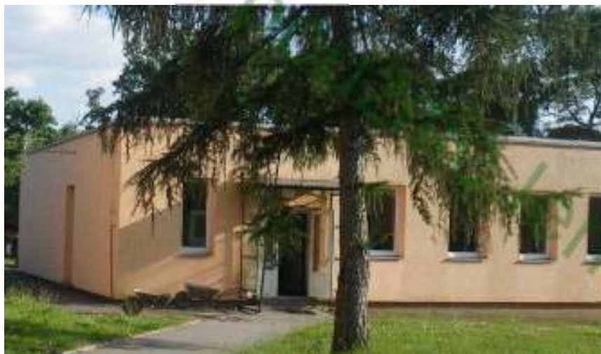
Radon corrective actions installed in 2013
